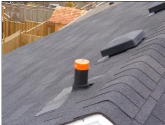
18. Plumbing stack is capped
