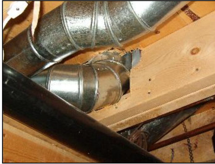
4. Double joist cut for ductwork
