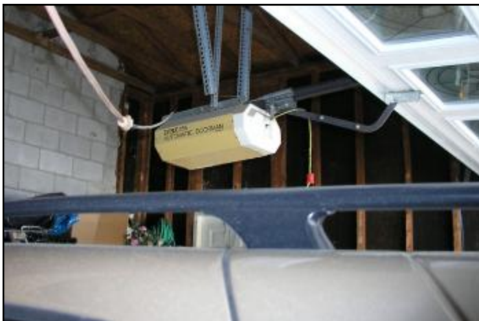
20. Extension cord for west garage door opener
