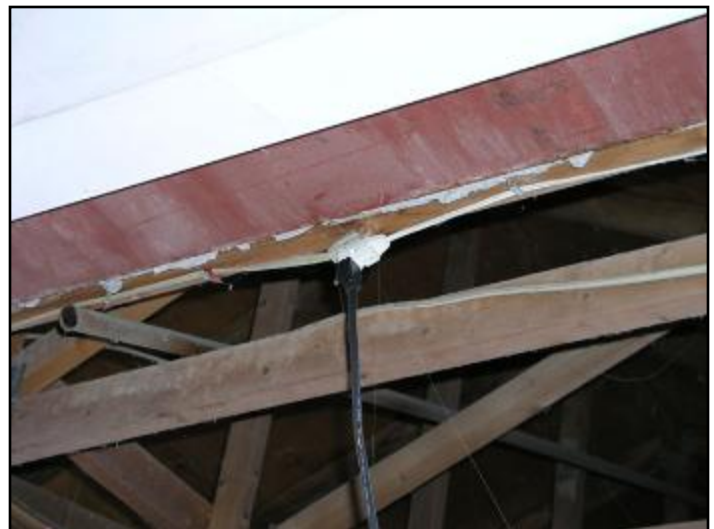
21. Extension cord for east garage door opener
