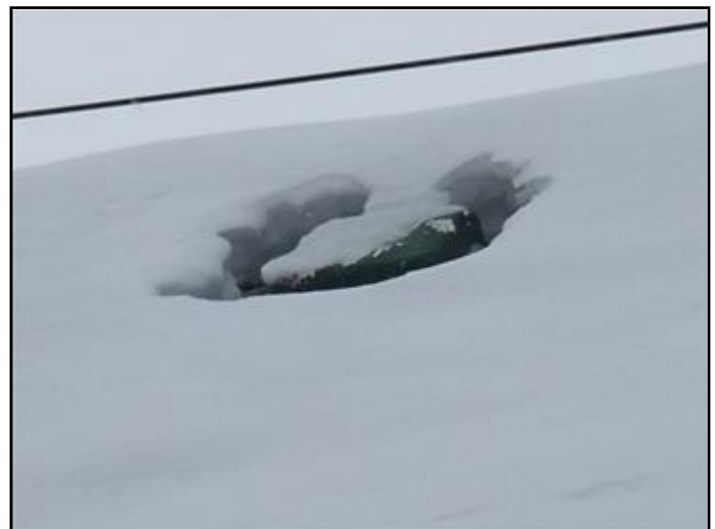
27. One only, roof vent visible
