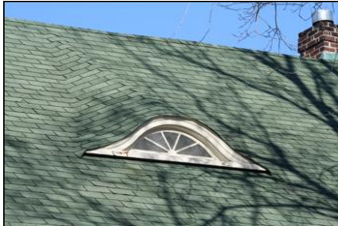
1. Asphalt roofing with decorative dormer
