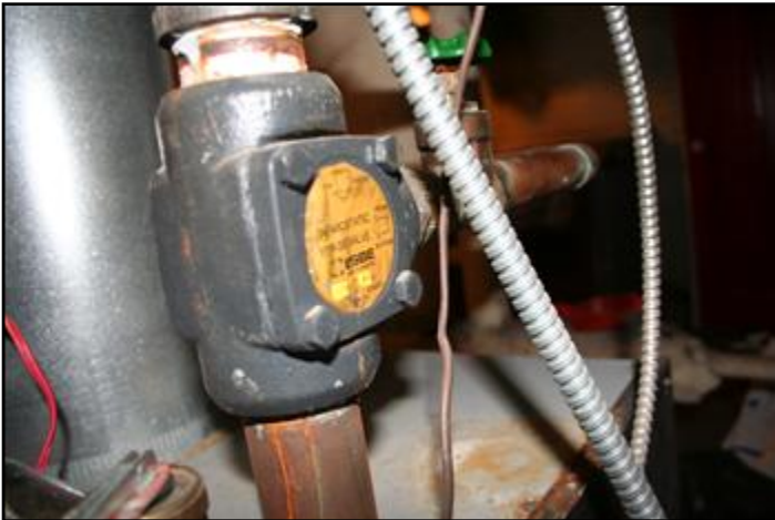
15. Thermostatic bypass valve
