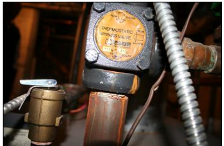
6. Thermostatic bypass valve
