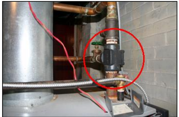
2. Thermostatic bypass valve
