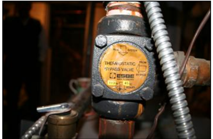
16. Thermostatic bypass valve
