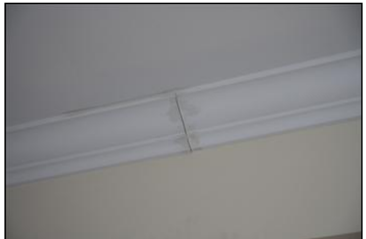
5. Living room crown moulding - west wall
