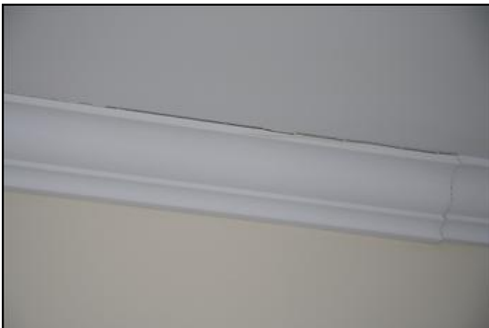
4. Living room crown moulding - east wall
