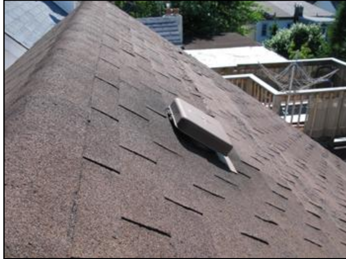
1. Asphalt shingles
