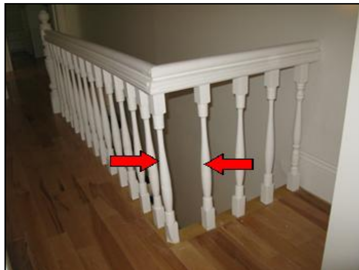
18. Wide spacing in railing
