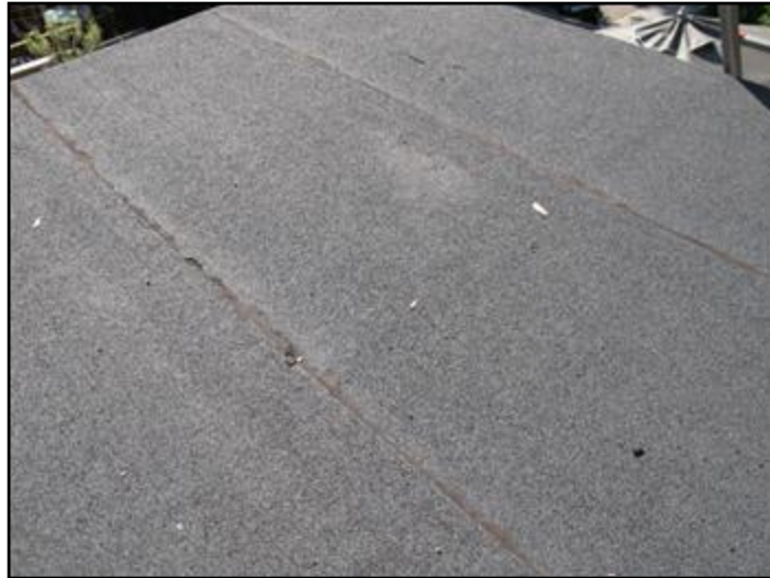
2. Flat roof at rear is in good repair
