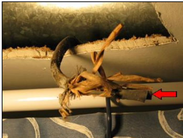
13. Apparently abandoned wire
