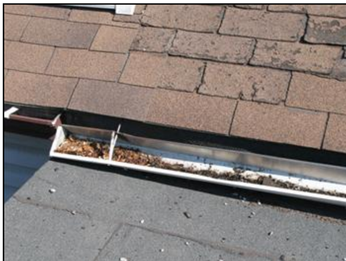
5. Loose gutter
